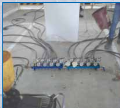
Underpinning with Patented Pre-Loading System
